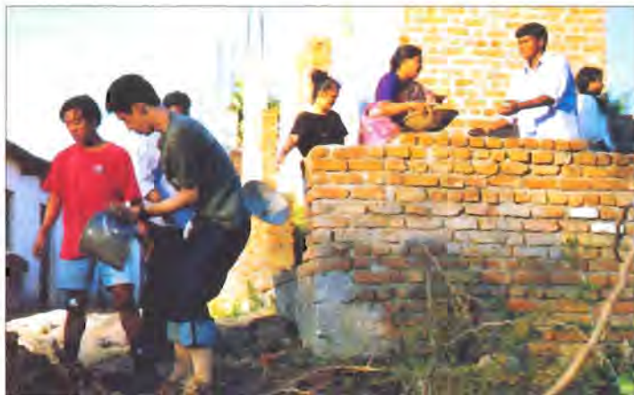
The RYS participants at work on the construction project
